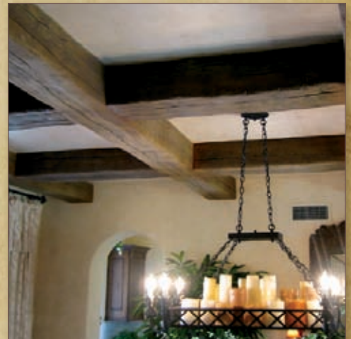
RUSTIC WITH CRACKS
